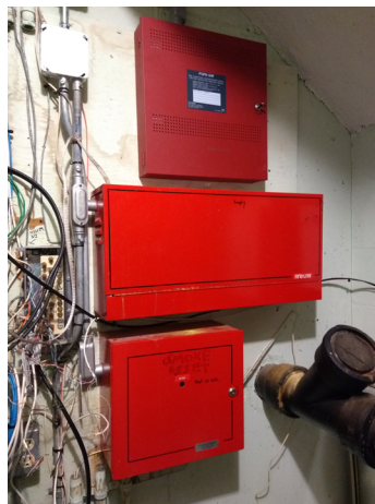
5. Update fire alarm system.
