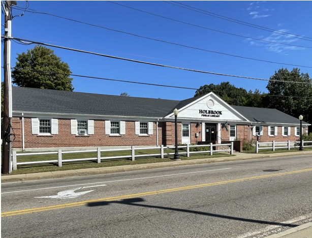
1. Front of building.
